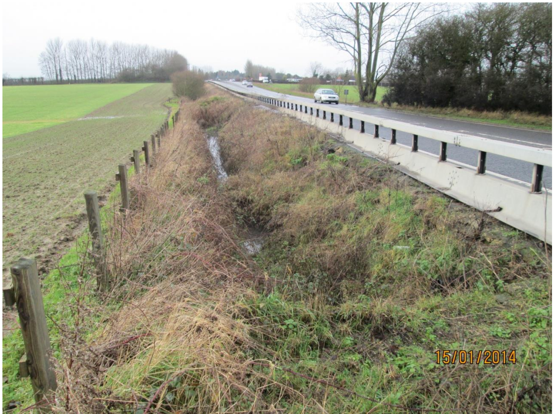
Photo 1 Looking along ditch with failure material in foreground and level with car
