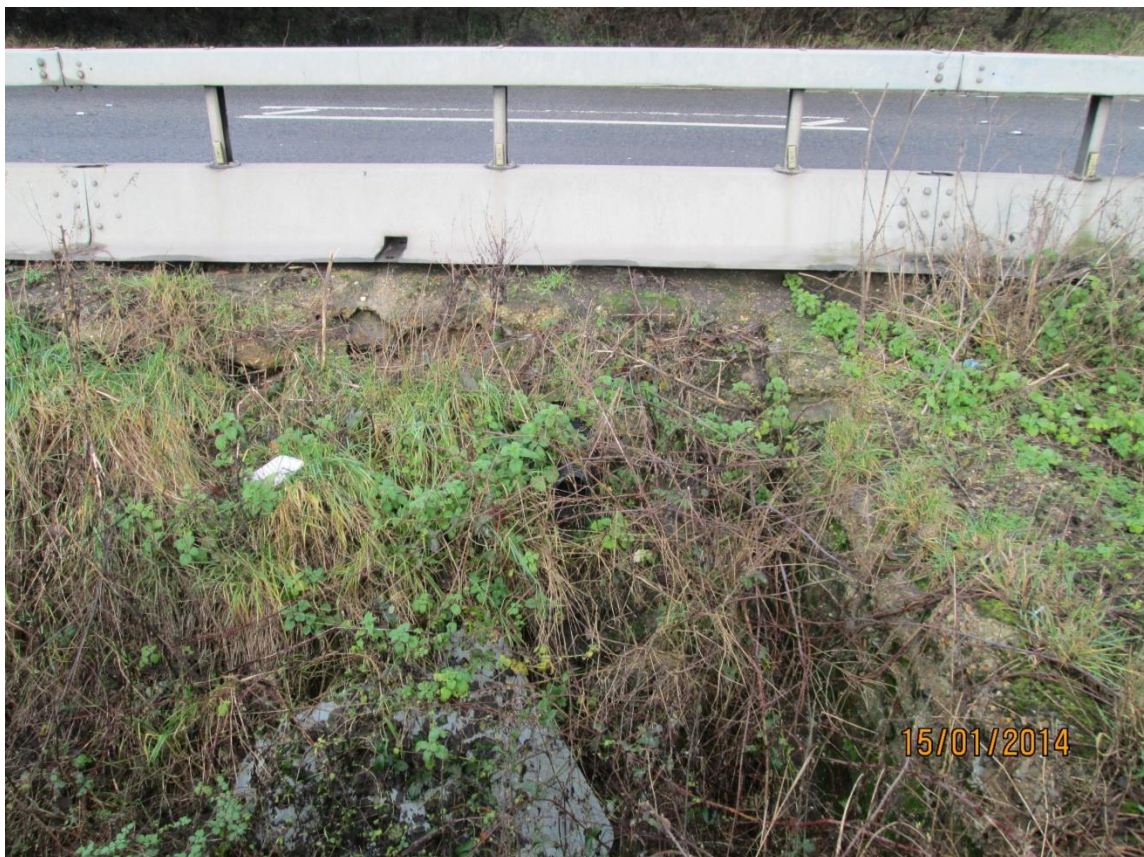
Photo 2 Area of failed material with black pipe visible through brambles – possible bag work repair on right
