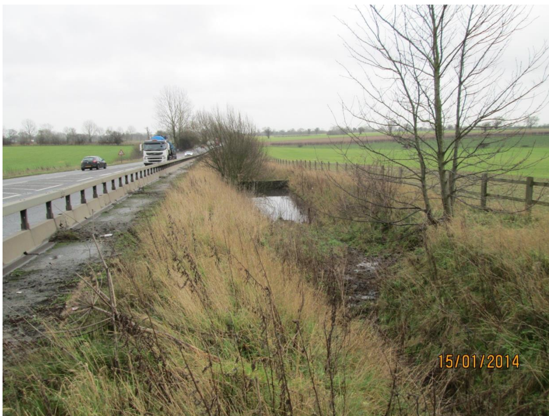
Photo 6 Ditch showing failed material in ditch base
