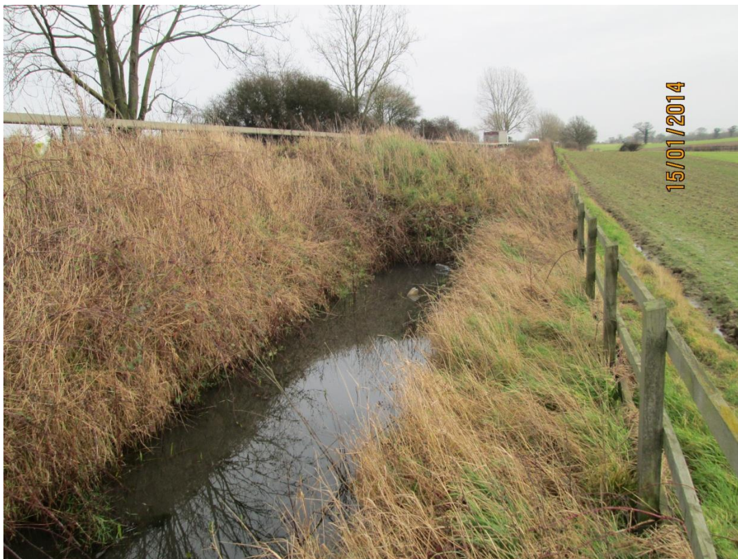
Photo 5 Ditch showing failed material in ditch base
