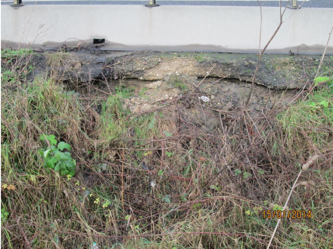
Photo 3 Area of failed material exposing depth of concrete under road pavement, possibly reflecting haunch repairs
