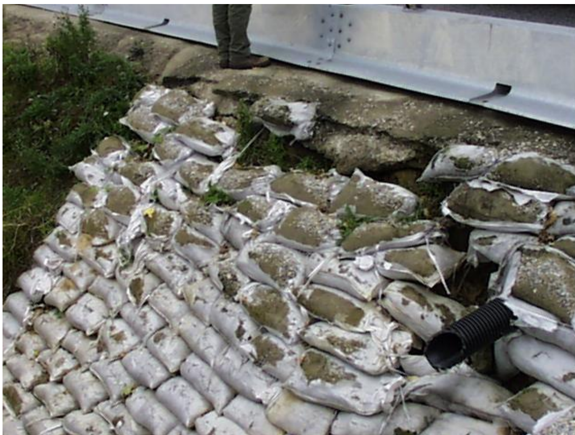
Photo 7 : 2004 inspection showing bag work with outfall pipe and varioguard in place
