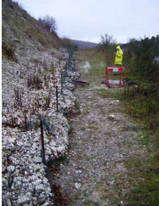
Figure 5 Ravelled material from a rock slope
