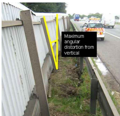
Figure 9 Measurement of angular distortion of a fence post
