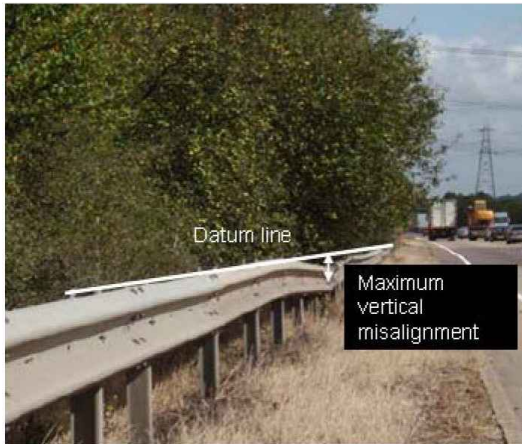
Figure 8 Measurement of vertical misalignment
